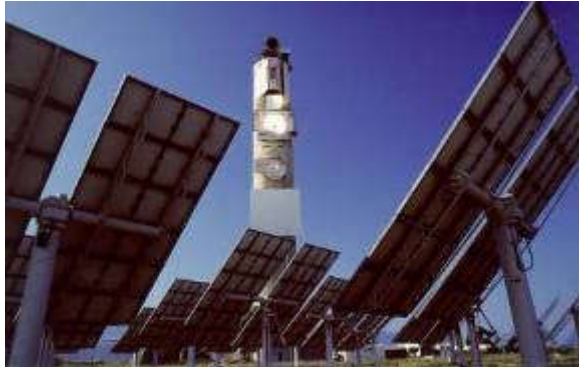
Solar thermal power plants
